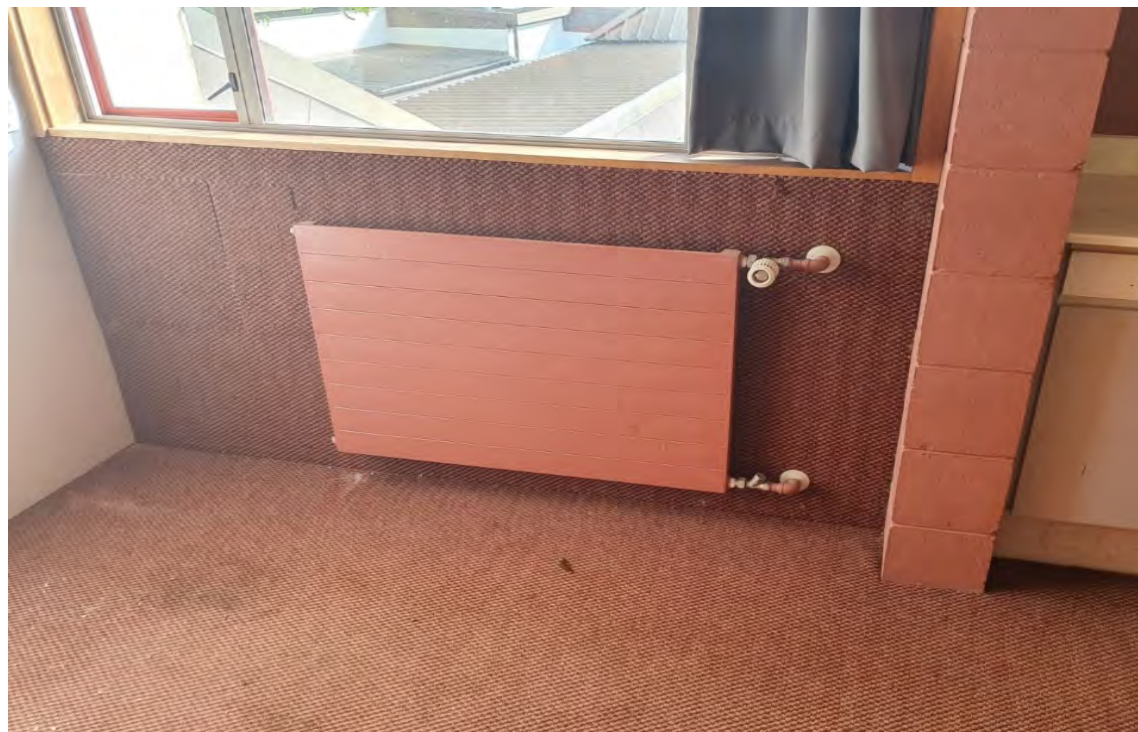
Figure 4 – image of a floor standing VRF indoor unit and existing radiator system in the barracks
