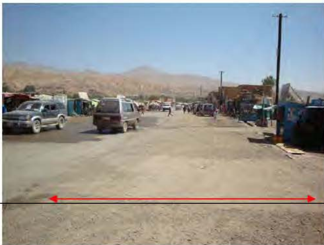
The Bamyan Bazaar Road needs to be sealed edge to edge.
