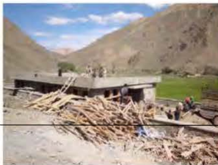
BHC under construction in Sayghan.
